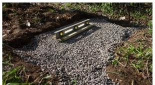
It is important that a honey bee hive is placed on level ground with good drainage. We started by selecting a southern facing location, excavating down about 4 inches, spreading coarse gravel for drainage, leveling, and placing large concrete blocks on which to install the hives.
